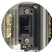
Example of internal 1-pole switch
