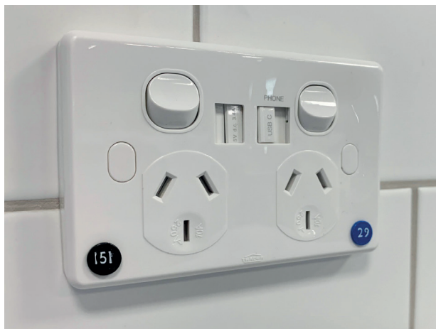
Fixed cover and fully shuttered Integrated USB charger.
