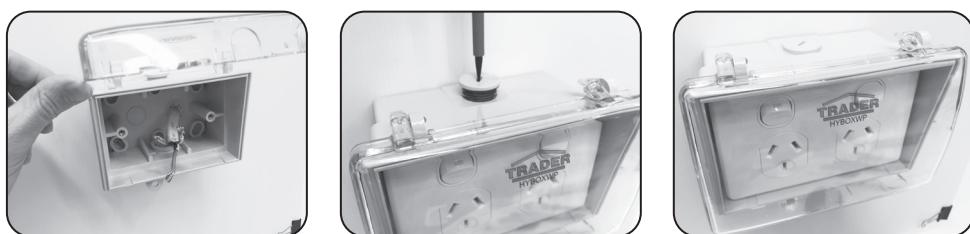
1. When installing the HYBOXWP ensure the product is mounted securely against the wall using the drill points in the covered recesses. Ensure the screw area is well sealed with silicone to protect the IP rating and apply internal screw caps.
